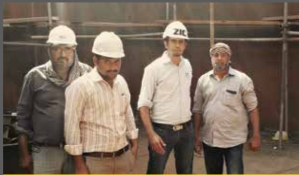
Inspection of Mechanical work taking place under the supervision of Third party inspector Mr. Ajmal Shah with the site engineer
