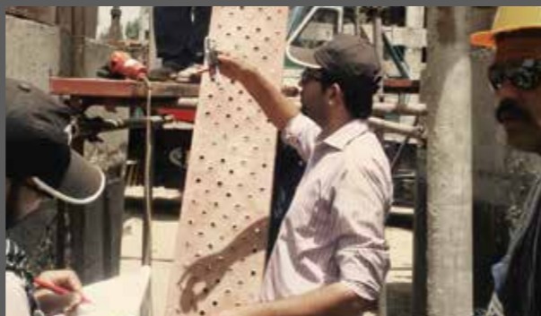
Nouman inspecting the bottom plate thickness of the tanks
