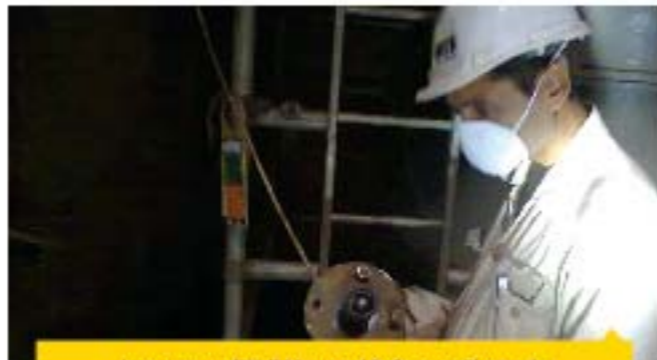
Inspection of Wall Mounted Reference Electrode
