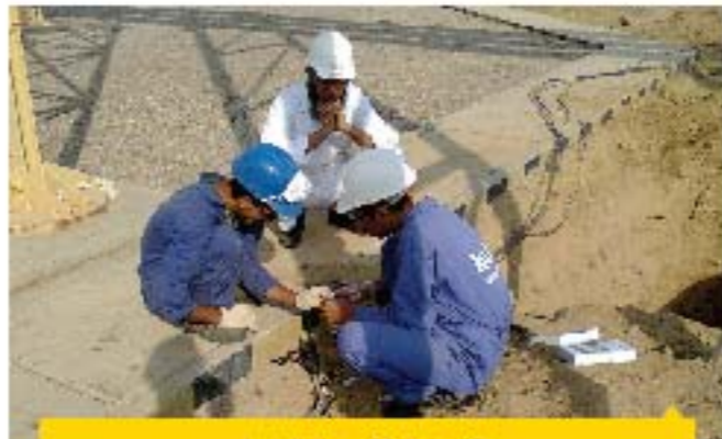
Installation of Splicing Kit
